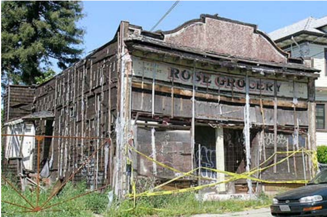
Eve of demolition, 2004.
